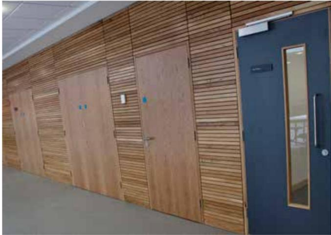
Store rooms doors using both lever handles and cylinder pulls. Where store rooms will be opened infrequently, cylinder pulls may be more appropriate and cost effective. In this specific example, the hardware chosen adds to the clean, flush, architrave free style of the project.
