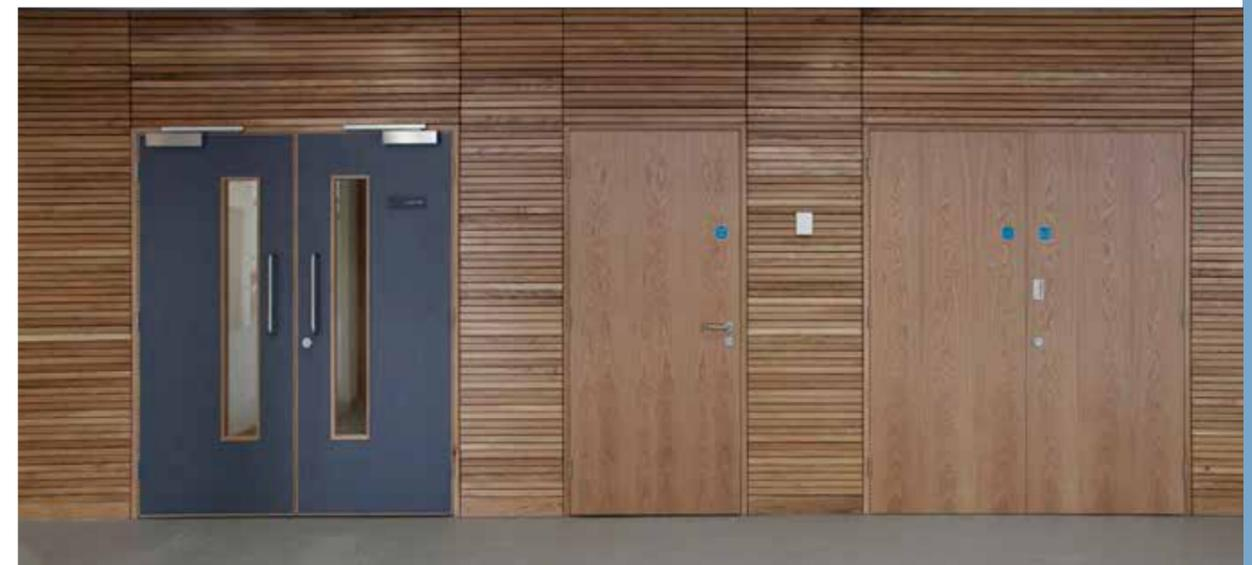
A combination of Formica Storm Grey laminate & American white oak veneered doors. Storm Grey laminate is complemented with exposed oak lippings, frames, architraves and glazing bead for circulation doors. Whilst contrasting crown cut, American white oak service and store room doors, act as a way finding feature for students and teachers.
