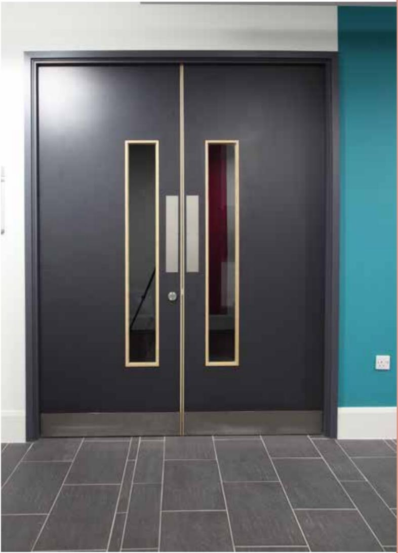
Vision panels allow students to view what is on the other side of the door and are an important safety feature, vital in preventing injury resulting from collision with opening doors
